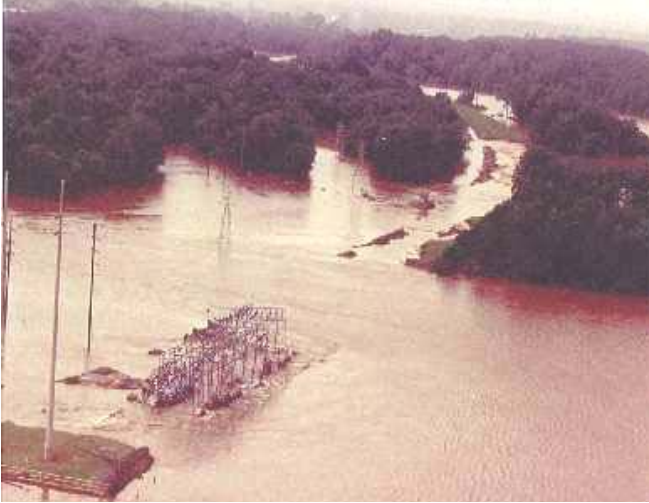
Company levee failure, Georgia, Sept. 14, Georgia Tech) 1994.
