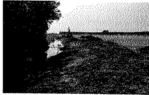
Construction start – widening the ditch and creating areas for wetland plants. Rock weirs along the wetland will help control water level and flow.
